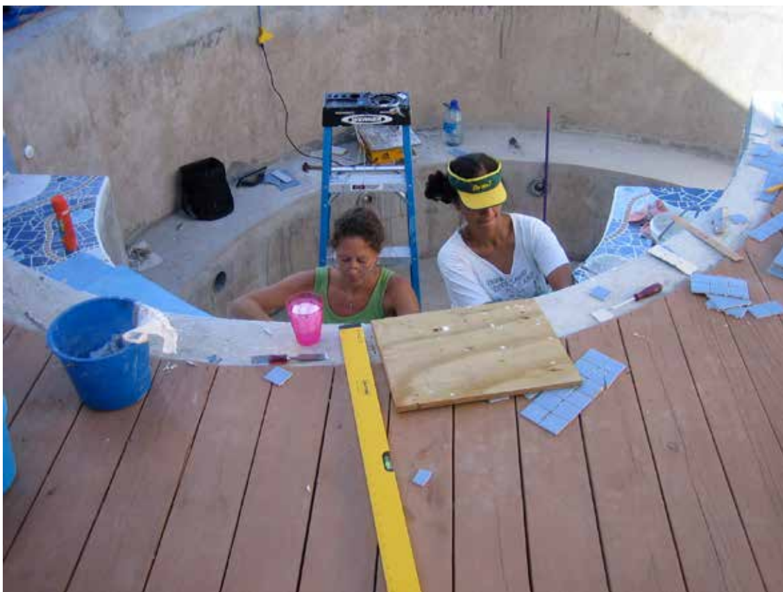
Completion of back wall mosaic
