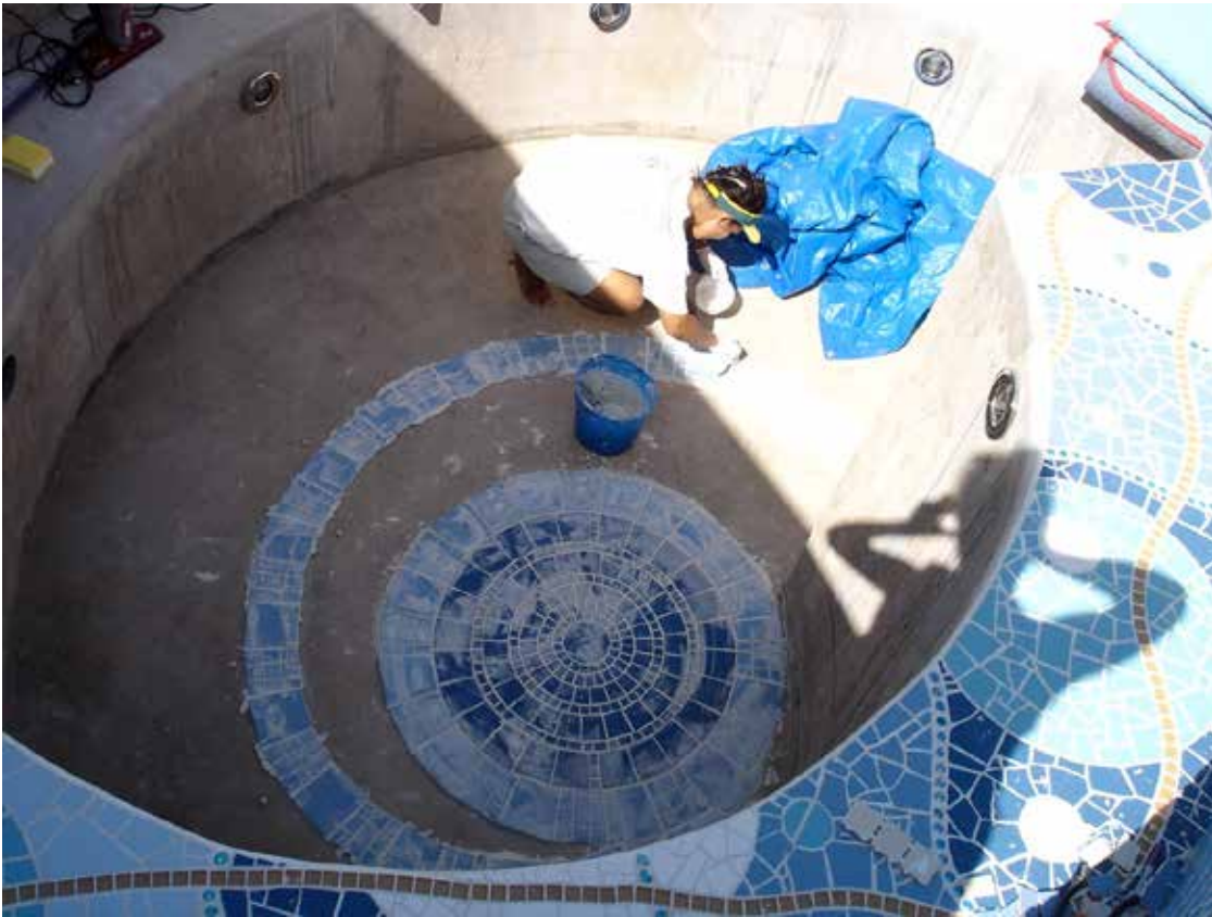
Installation of bottom graphic
