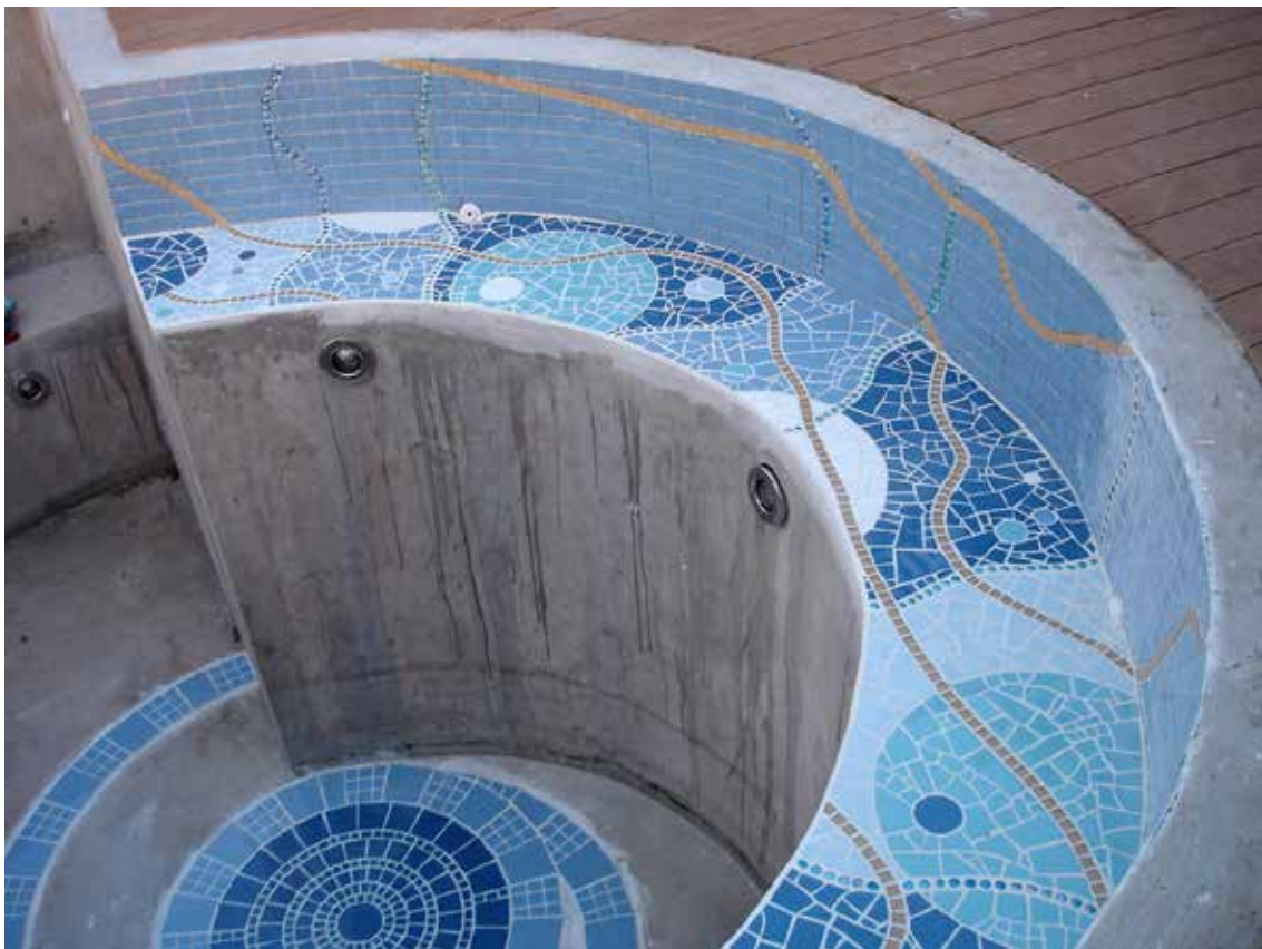
Completed mosaic prior to final wall grouting and pool finishing by contractor
