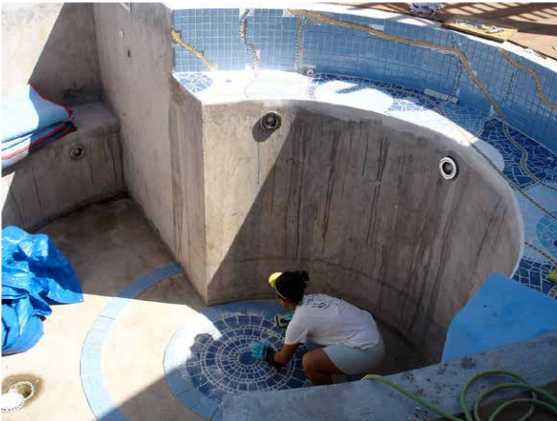
Completion/grouting of bottom circle and
